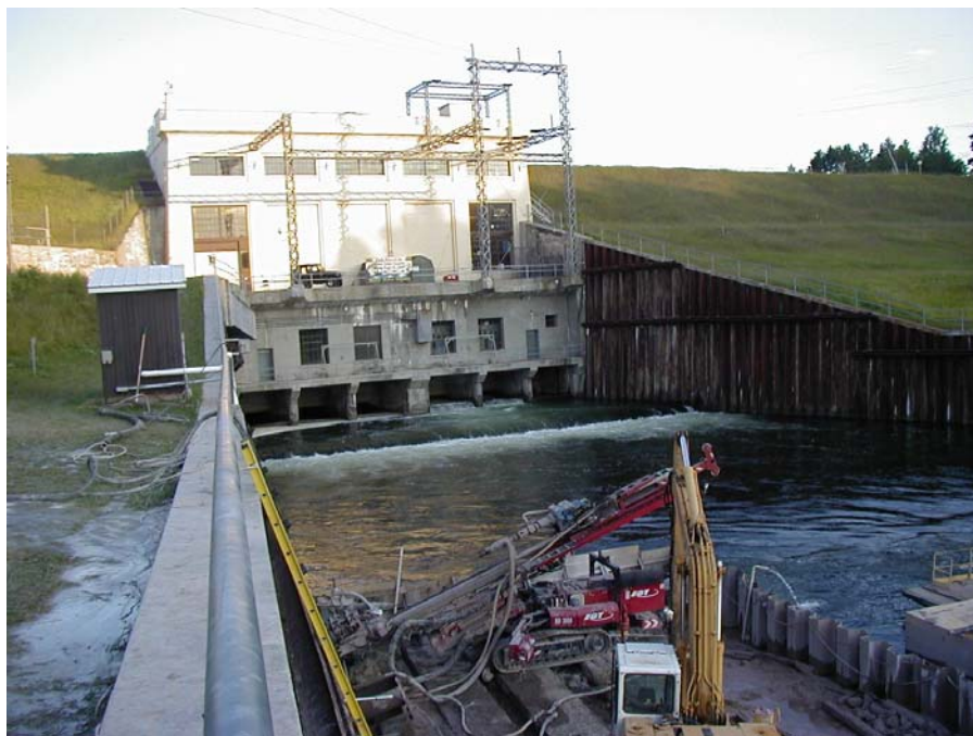
Figure 1. Downstream face of Hodenpyl Dam, showing right downstream retaining wall on left.
