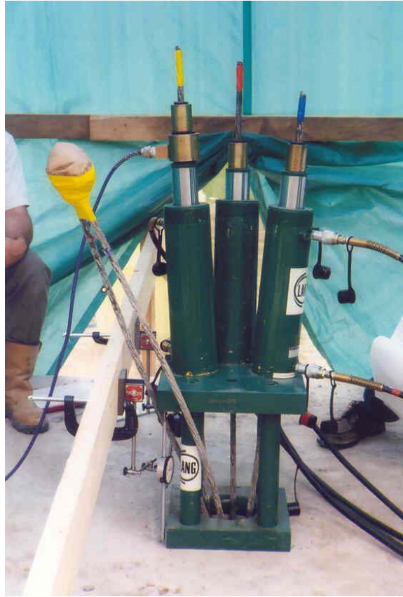
Figure 5. Sacrificial test anchor stressing jack.
