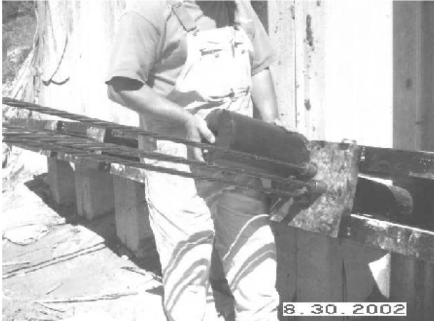
**FIG. 9.** Detail showing the anchorage elements. The strands are about to be cut and covered with the grease-filled housing.
