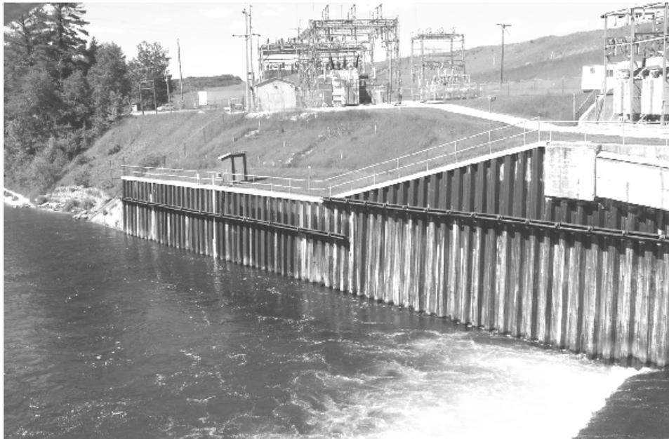
**FIG. 1.** View of the tailrace channel and east retaining wall. Note the existing tiebacks installed in 1996. The sheetpiles were also added in 1996 as a facing and do not penetrate below the footing
