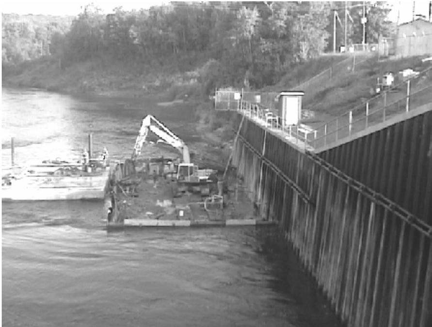
**FIG. 7.** View of the site during installation of the SBMA elements. a sheet piling cofferdam provided a dry working area below the tailrace water level. Note service barge on the left.
