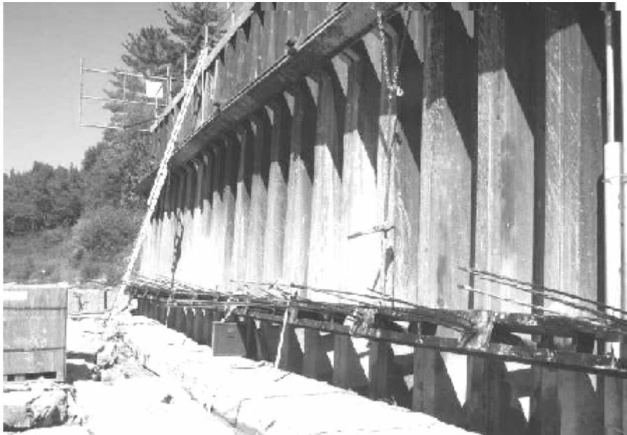
**FIG. 8.** View of the wall at near completion of the installation of the SBMA elements near the bottom of the wall. The strands are to be saw-cut and covered. The old tieback installation is visible near top of photo.
