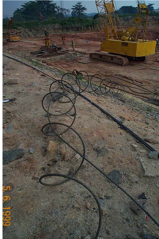
Photograph 2. Extracted strand of a removal anchor.
