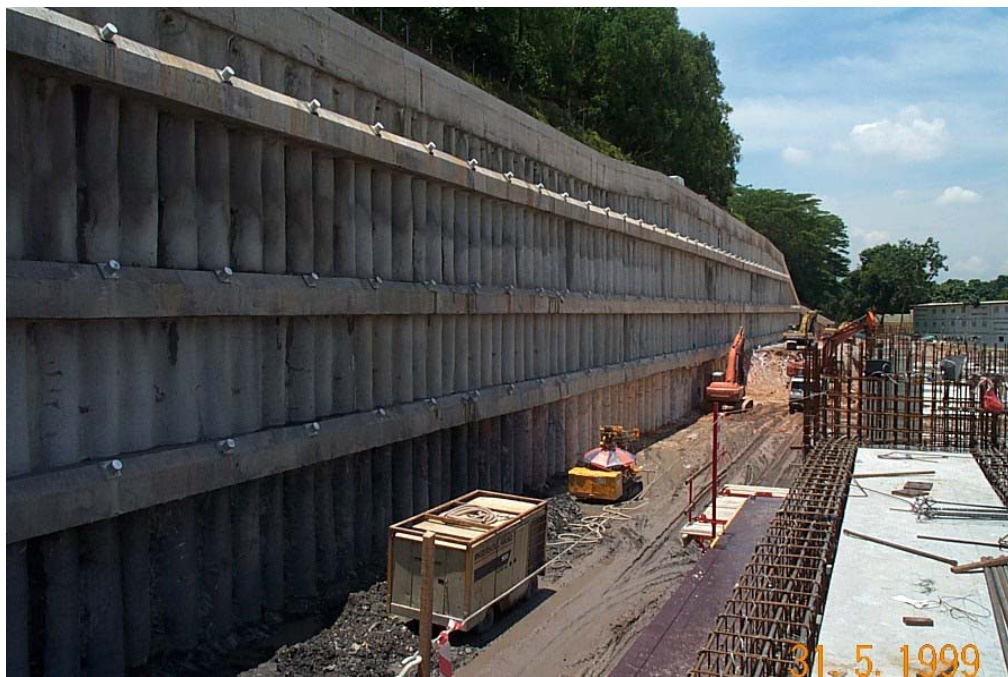
Photograph 4. 150-tonne working load anchors allowed the original number of 80-tonne anchors to be reduced by half.
