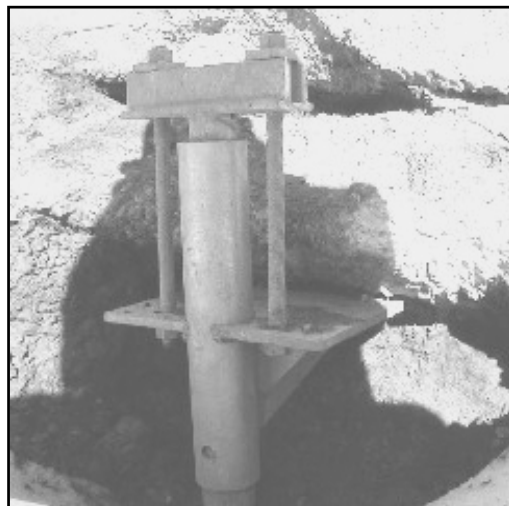
FIG. 9. Pre-manufactured Bracket that can be used for Micropile Underpinning Applications
